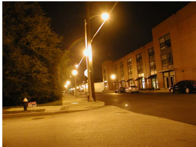
Sidewalk Illumination – Existing Conditions
